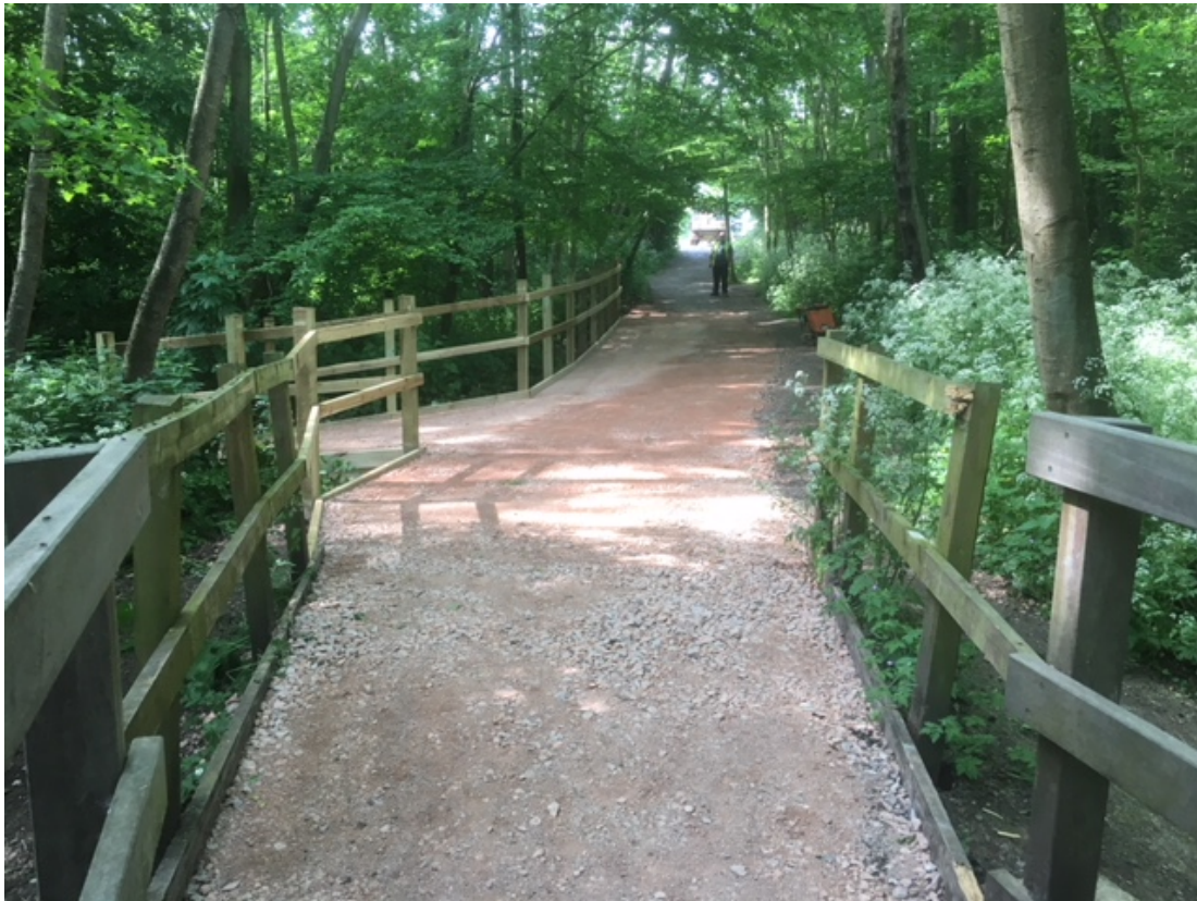
Footpath Repairs – Peatmoor
