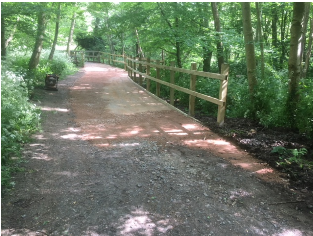
Footpath Repairs - Peatmoor
