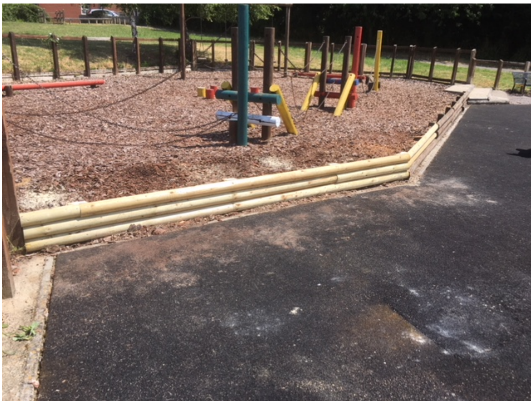
New Edging Boards and Topped up Bark
